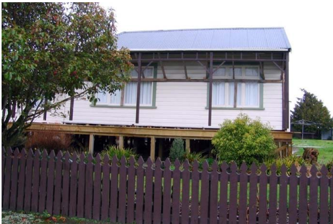
Figure 8. Residential building on raised foundations.
