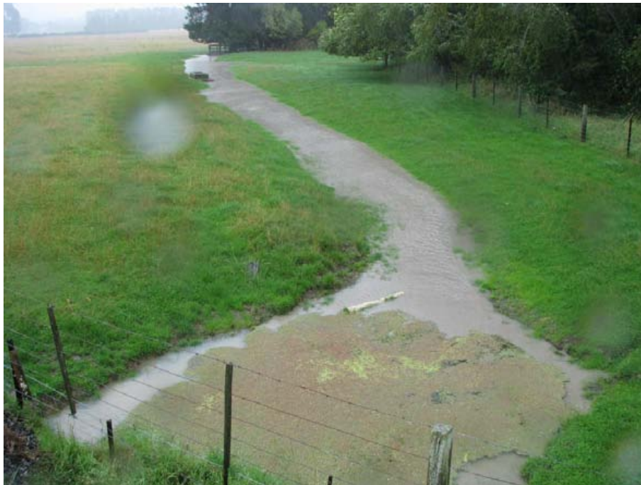
Figure 6. Rural floodway corridor near Back Road draining surface runoff during a rainfall event in February 2012.
