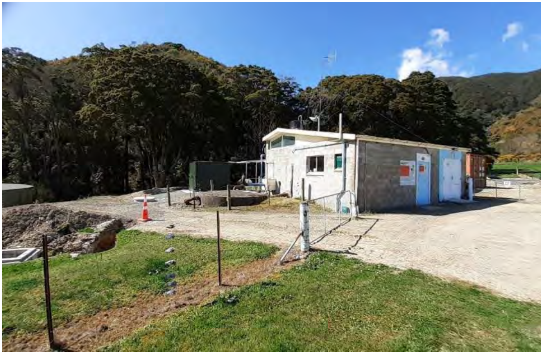
Figure 5-69 The Tapanui Water Treatment Plant
