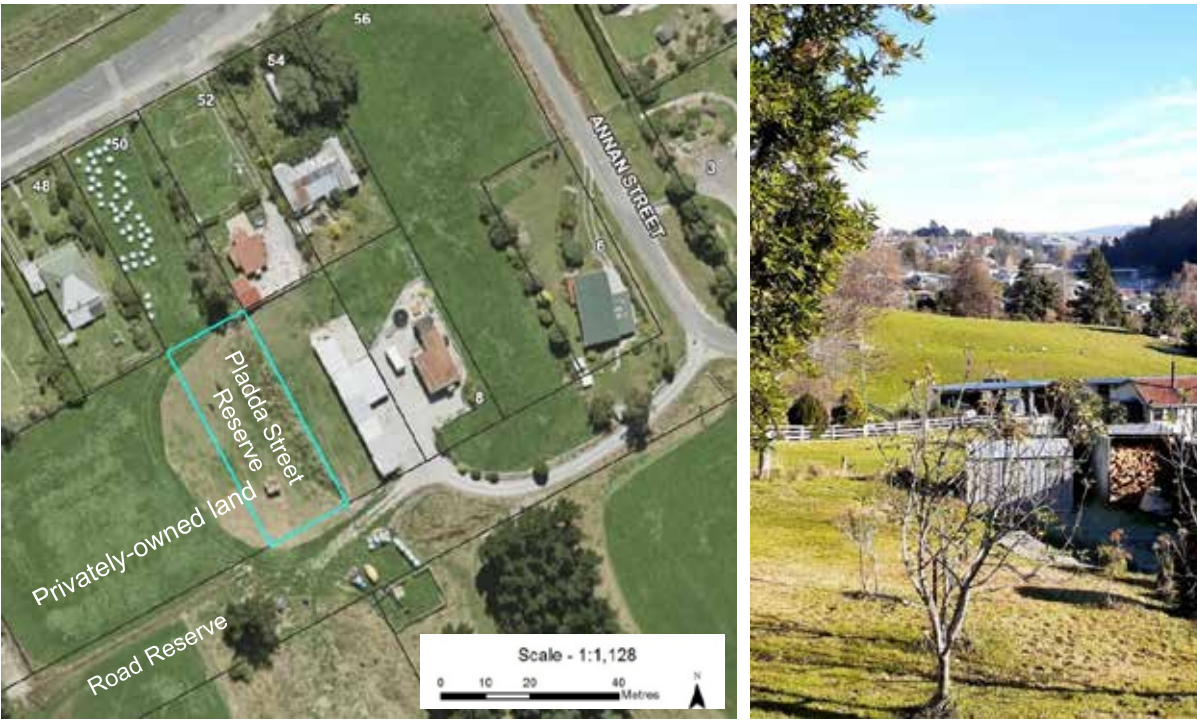
Figure 4-20 Left: Aerial photo, showing the boundary of the Pladda Street Reserve. Right: View towards the reserve from Annan Street.
