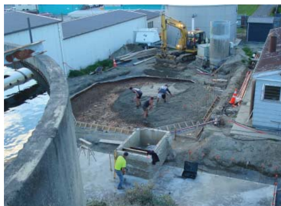
Balclutha water treatment plant upgrade
