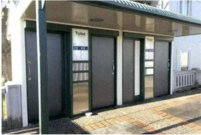
Refurbished Toilets at the Balclutha Information Centre
