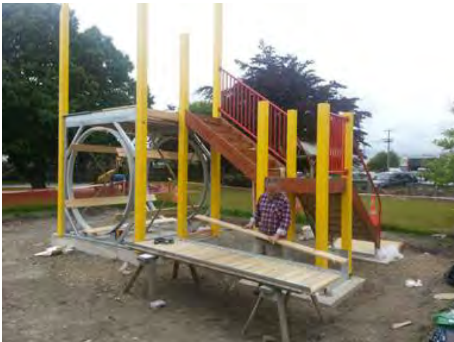
New playground equipment in Balclutha under construction
