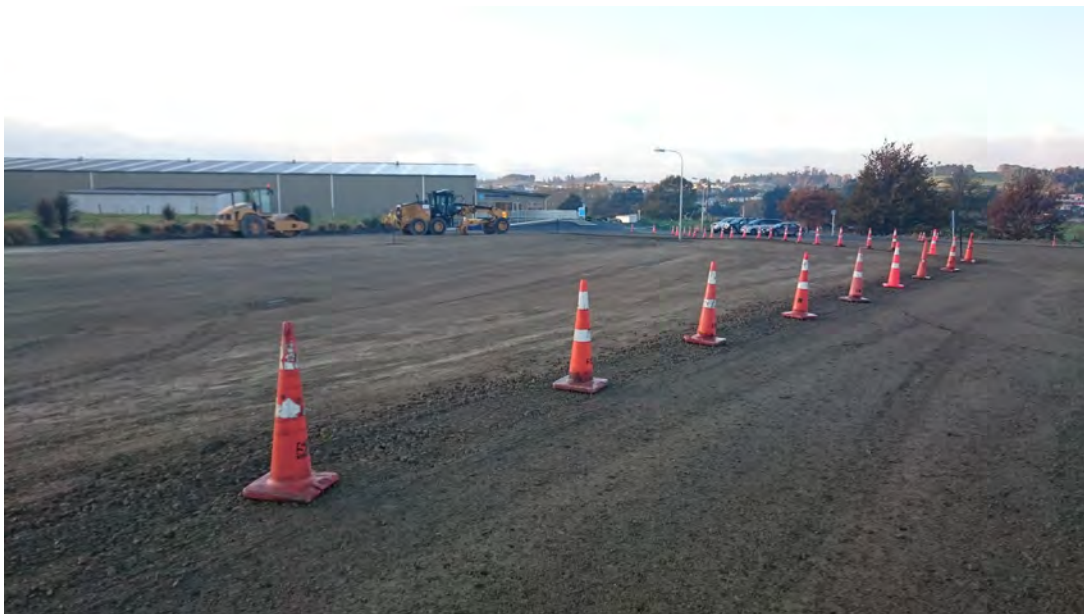
Sealing getting underway for Cross Recreation Centre Carpark
