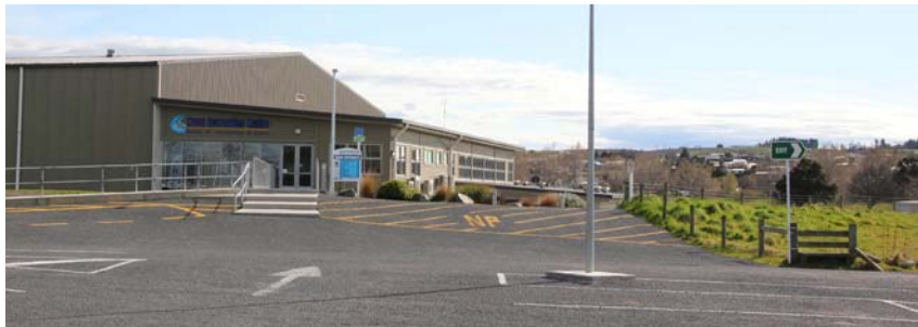
The end result of sealing at the Cross Recreation Car Park
