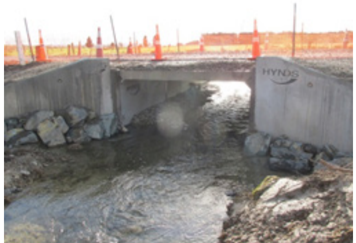
Construction of Bridge 406 - Mill Road in West Otago
