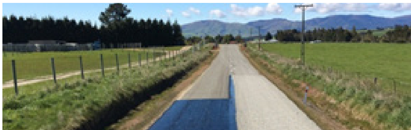
Resealing in progress on Shanks Road in West Otago
