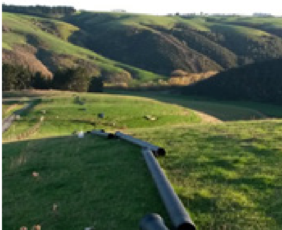
Waitahuna treatment plant rising mains pipes ready for placement
