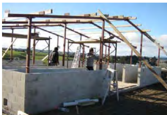
The new Balclutha Pound under construction
