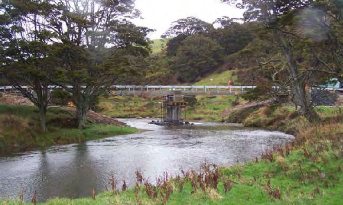
Replacement Tawanui bridge, June 2011
