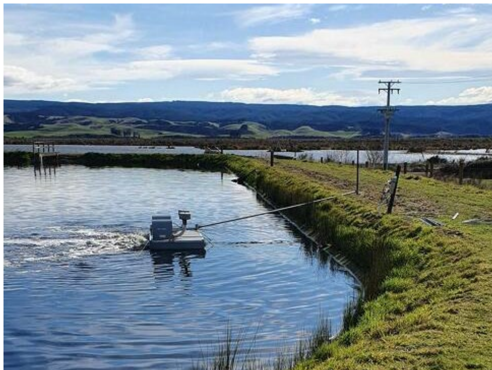
Aerator at Waihola Pond
