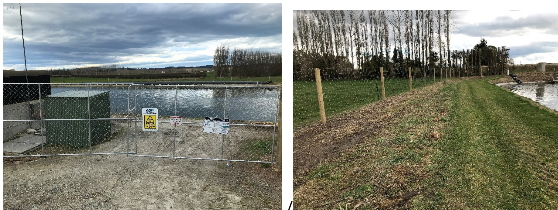
Stirling WWTP 1.8m deer fencing
