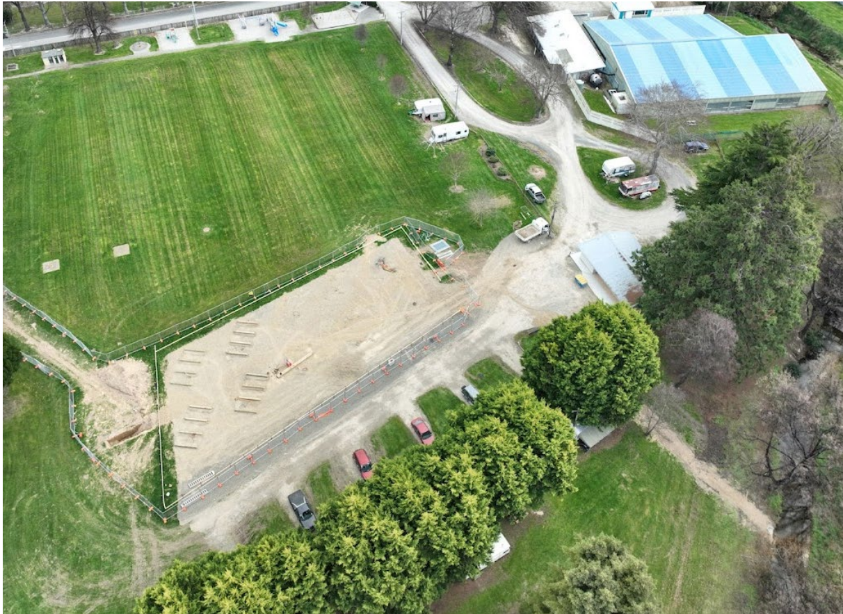
Figure 3-1 Aerial view of Taylor Park in September 2023 showing earthworks and foundations in place, in preparation for the placement of the first four cabins.
