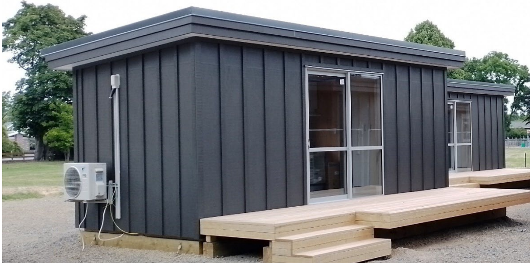
Figure 2-3 Cabins currently located at Taylor Park
