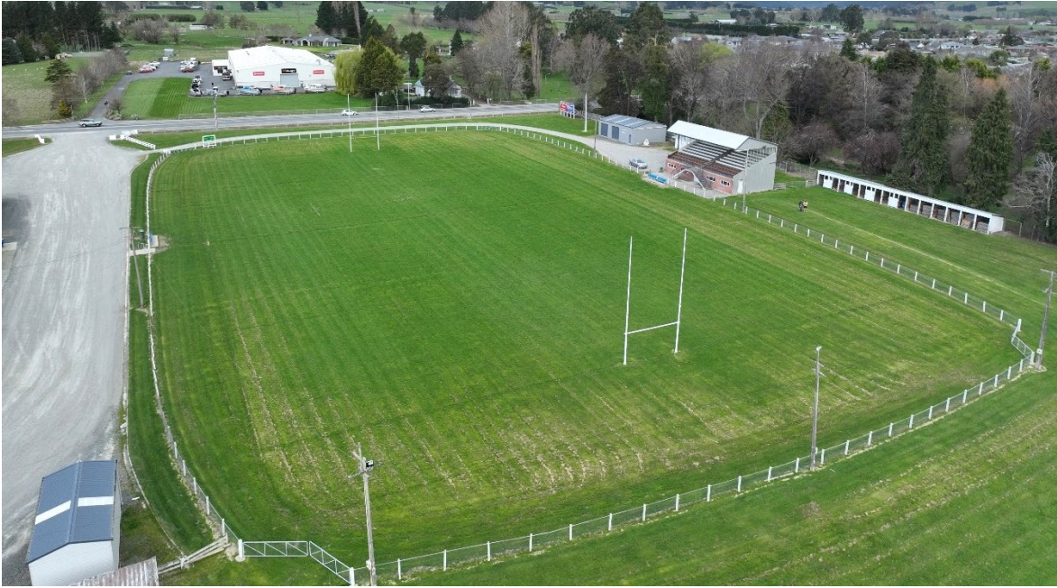
Figure 6-5 Aerial view of the Tokomairiro showground.
