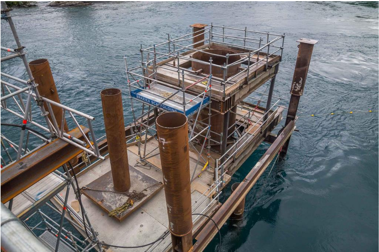
Figure 7: Example of Pile setup
