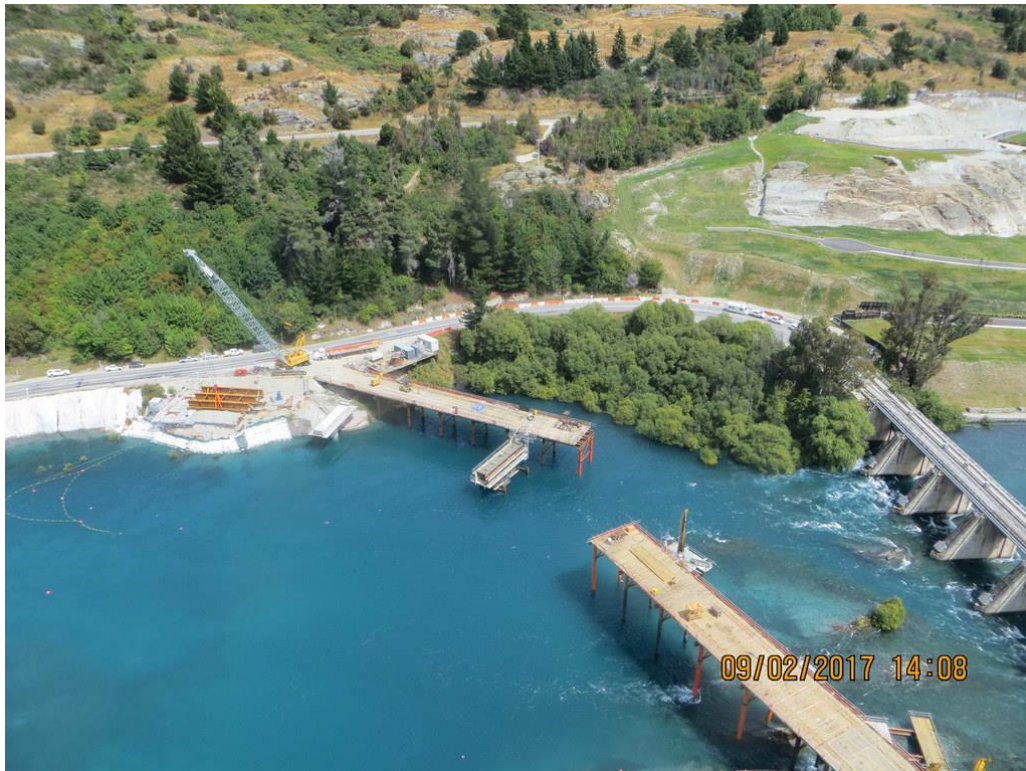
Figure 6: Photograph of temporary platforms - Kawarau Bridge
