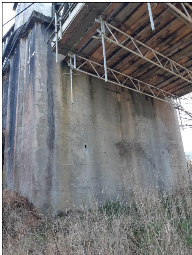
Figure 28. View looking north west of the Beaumont Bridge west abutment
