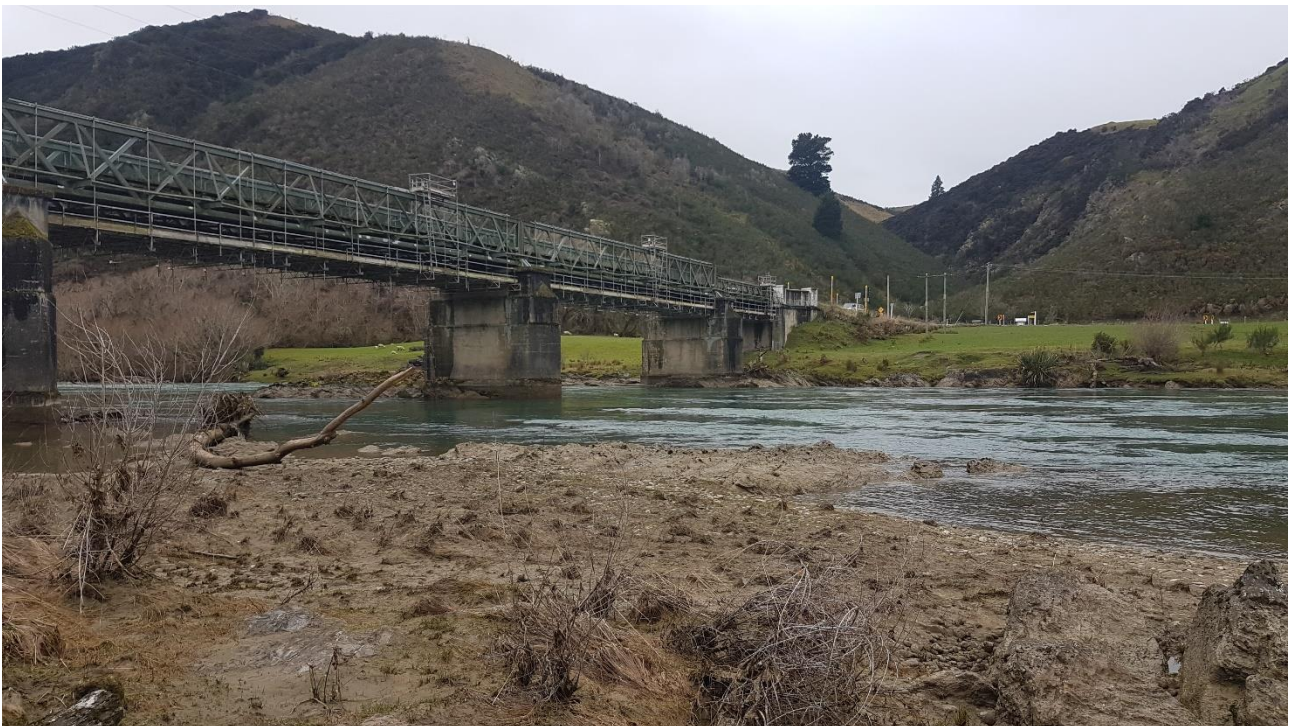
Photo 6: Eastern bank and existing bridge viewed from western bank
