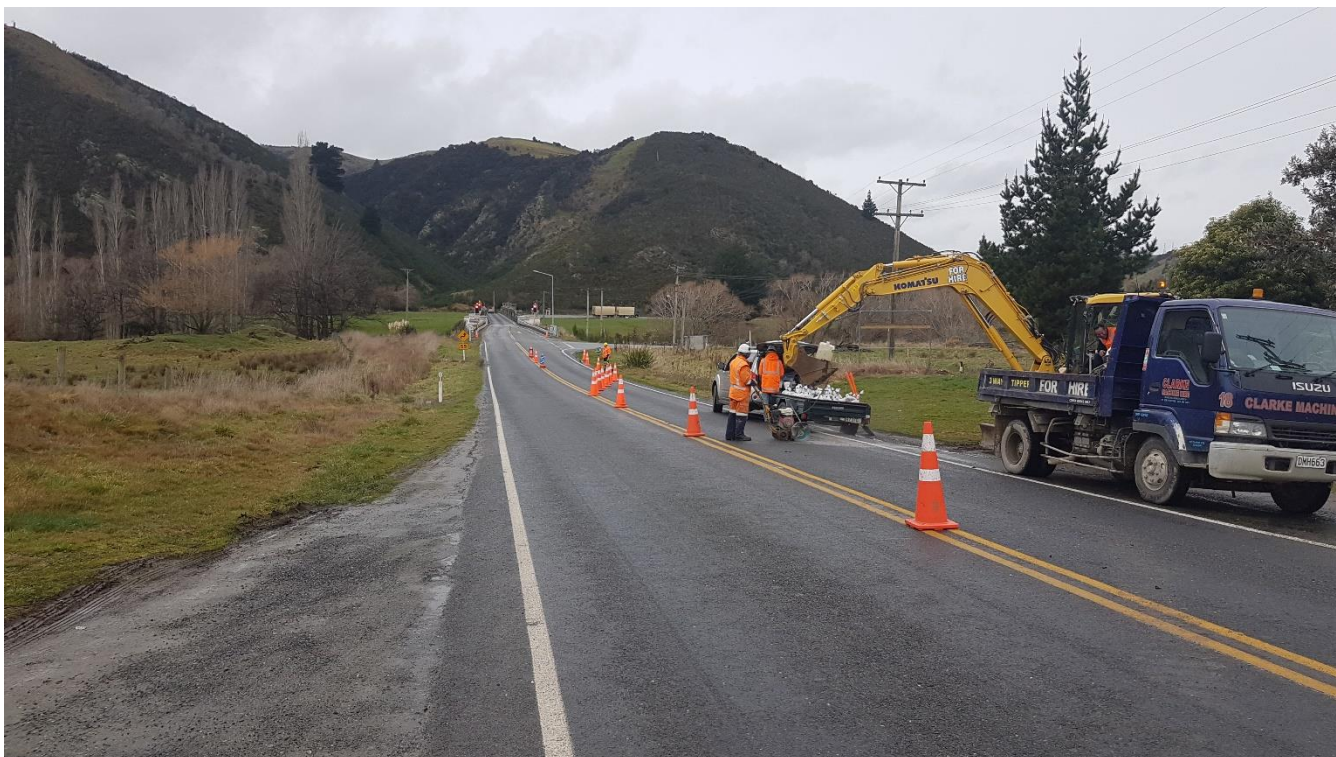
Photo 10: SH8 western side towards existing bridge
