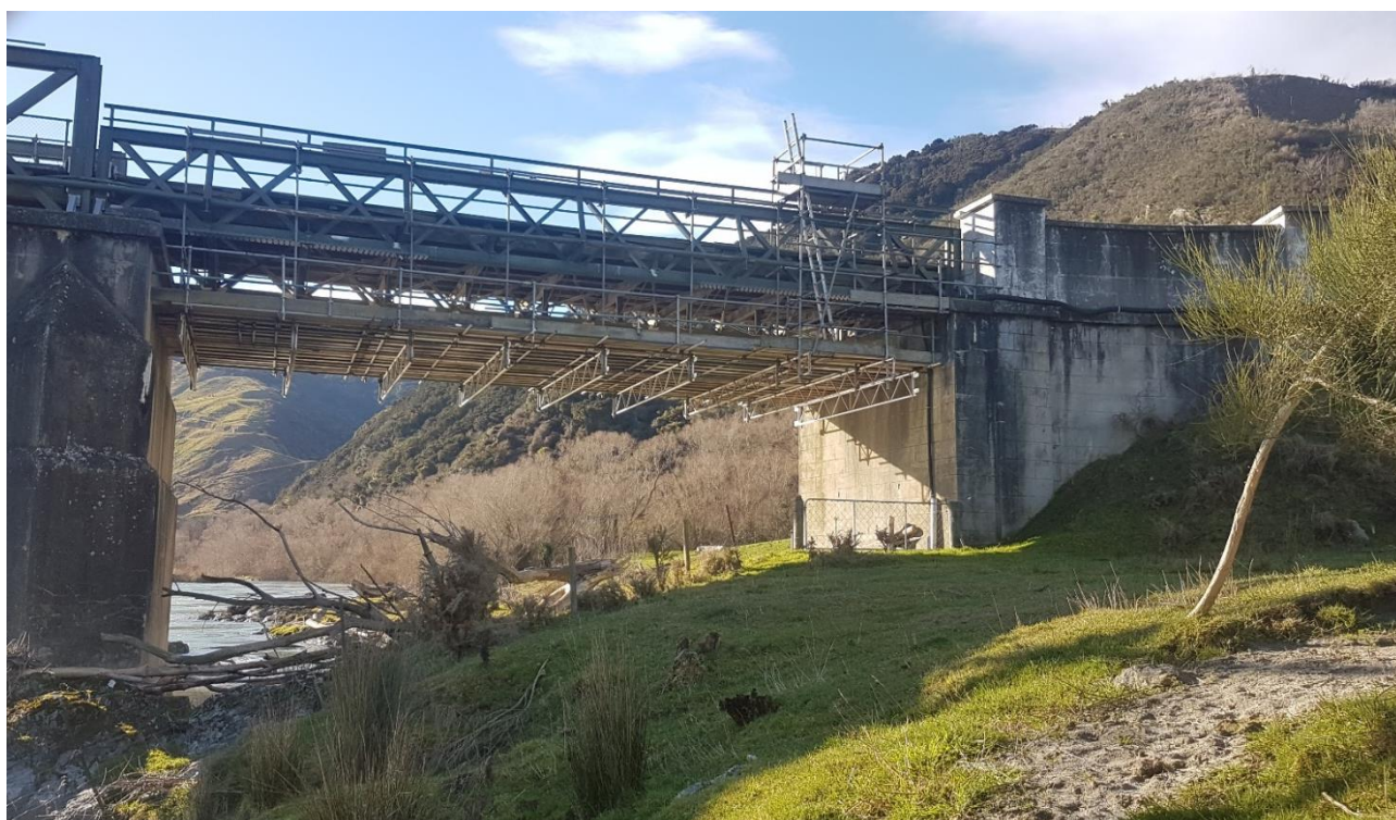
Photo 4: Eastern abutment of existing bridge
