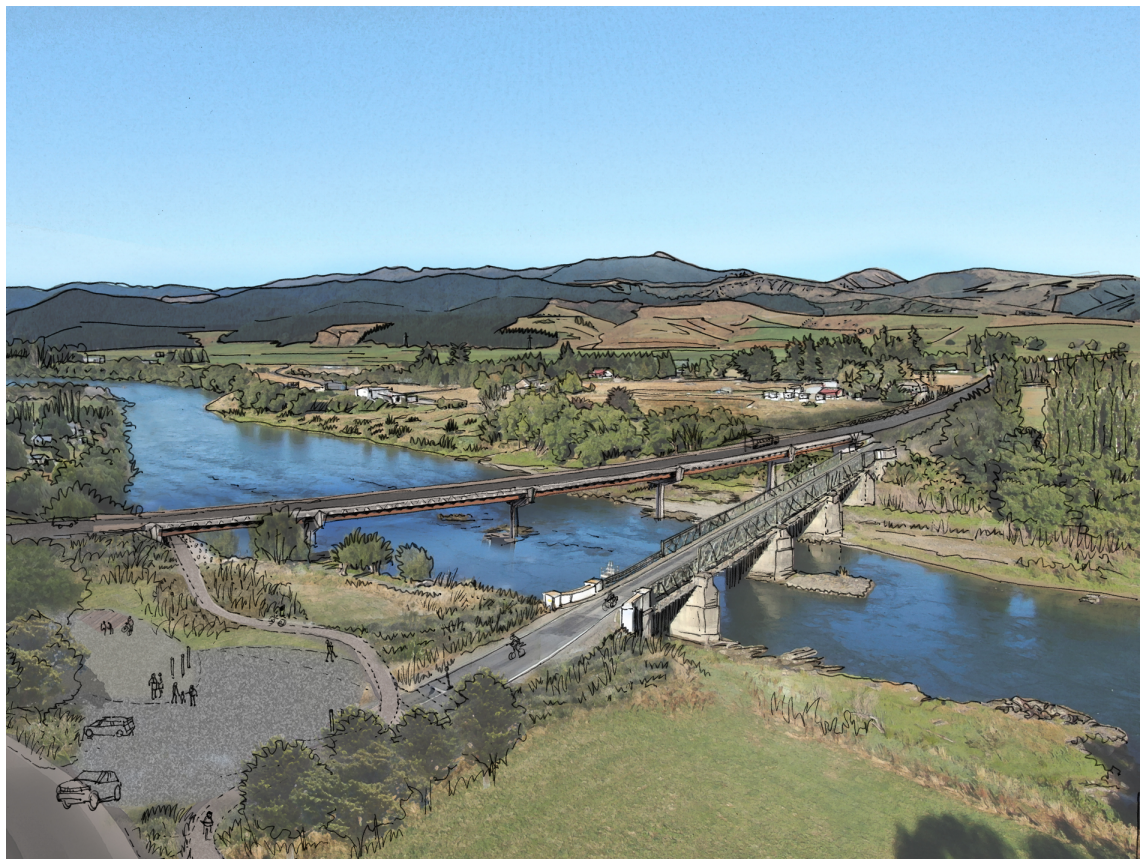
Figure 1 Artists impression of the new State Highway 8 bridge over the Clutha River at Beaumont, looking downstream showing the existing bridge in the foreground.
