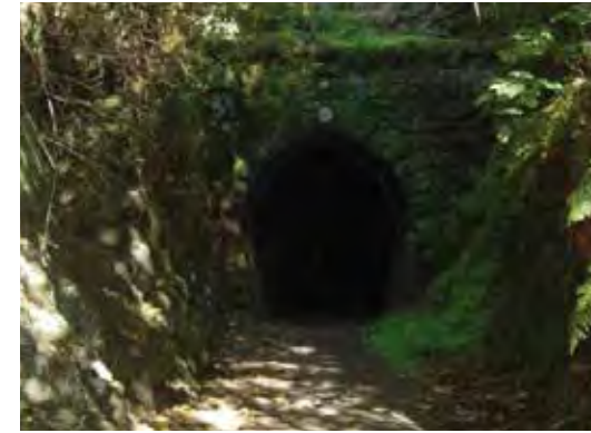
Old railway tunnel
