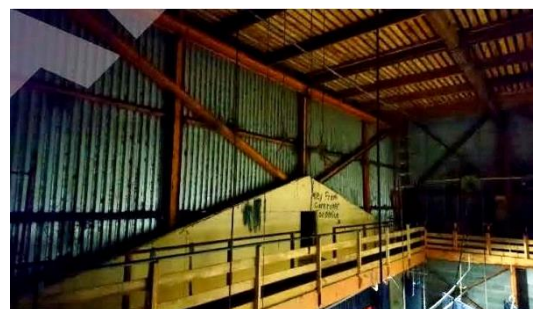
Steel work of 'front' wall.
