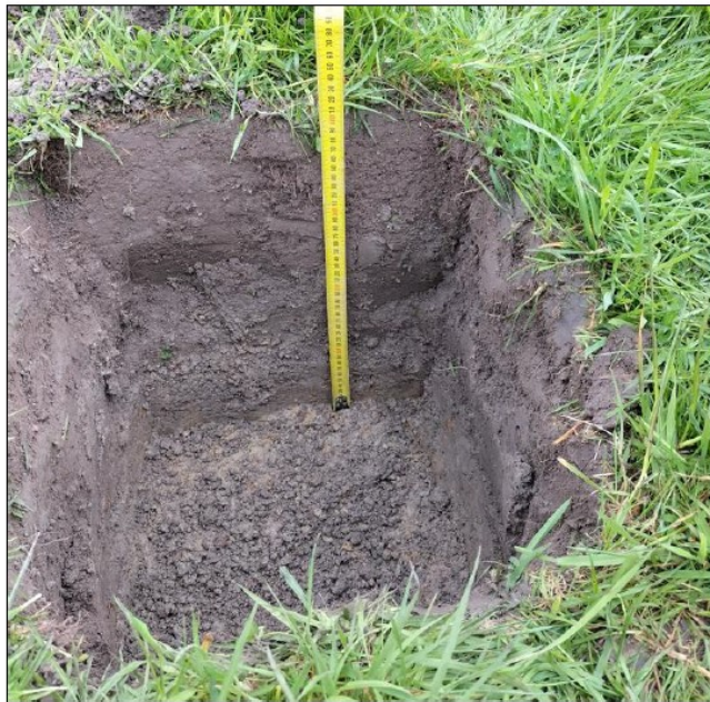
Figure 8.0: Excavated Test Pit
