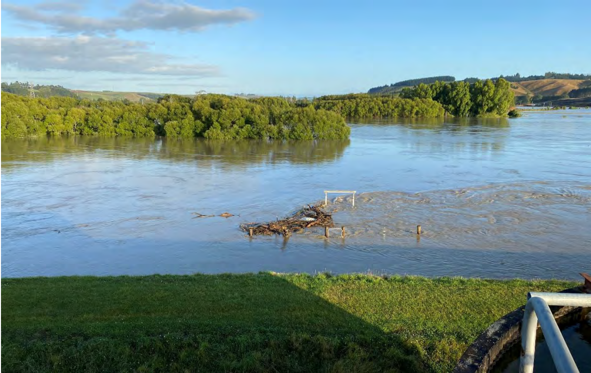
Figure 3-1 Balclutha Water Treatment Plant intake, during a flood event in February 2020 Flood (Source: CDC).
