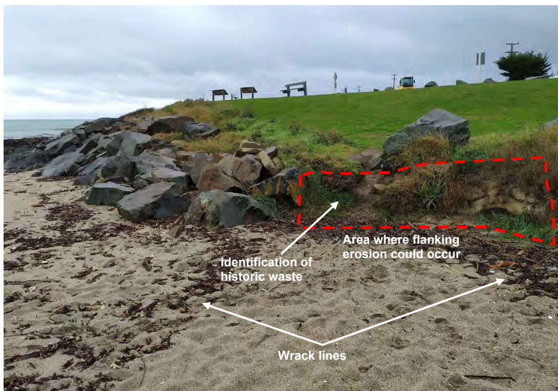
Figure 3-6 Northern edge of the rock embankment indicating where flanking erosion could occur. May 2021 (Source: GHC)
