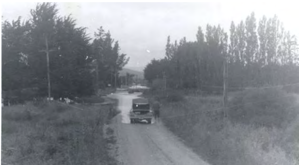
Figure 5-9 Road inundation, due to flooding in the Waitahuna River, January 1966 (source: ORC).
