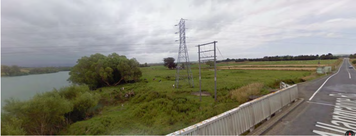
Figure 5-7 View of infrastructure and farm land on the true left bank of the Clutha River at Clydevale. Source: Google Street View
