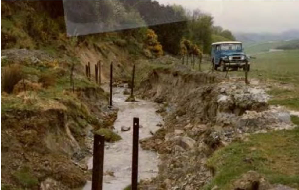
Figure 5-10 October 1978 Hunt Road Creek, Lawrence, showing streambank erosion. Source: ORC.
