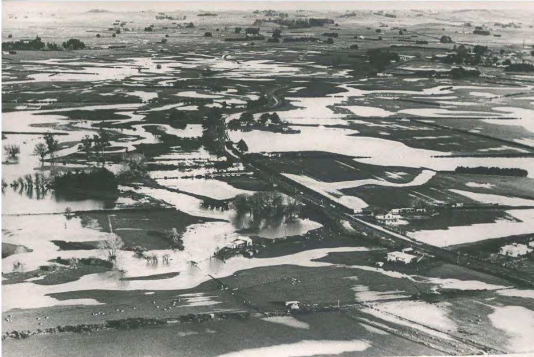
Figure 3-6 Flooding of SH1, near Milton in 1987 (source: Hocken Snapshot collection, University of Otago).
