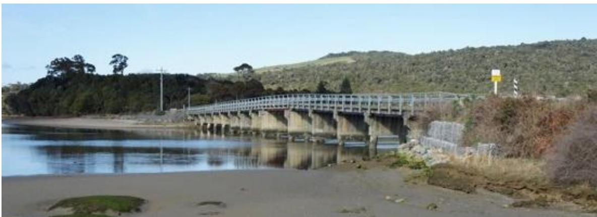
Figure 3-3 The Tahakopa River Bridge at Papatowai (October 2019, Source: GHC).
