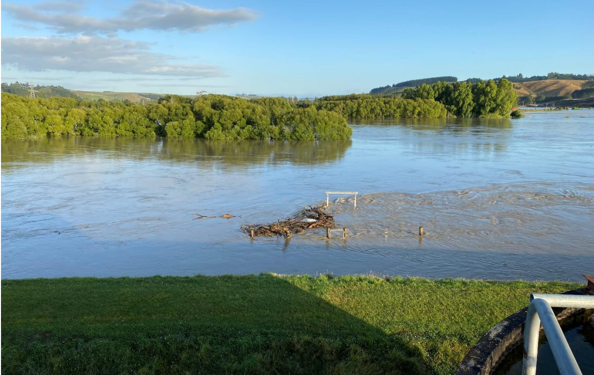
Figure 3-1 Balclutha Water Treatment Plant intake, during a flood event in February 2020 Flood (Source: CDC).
