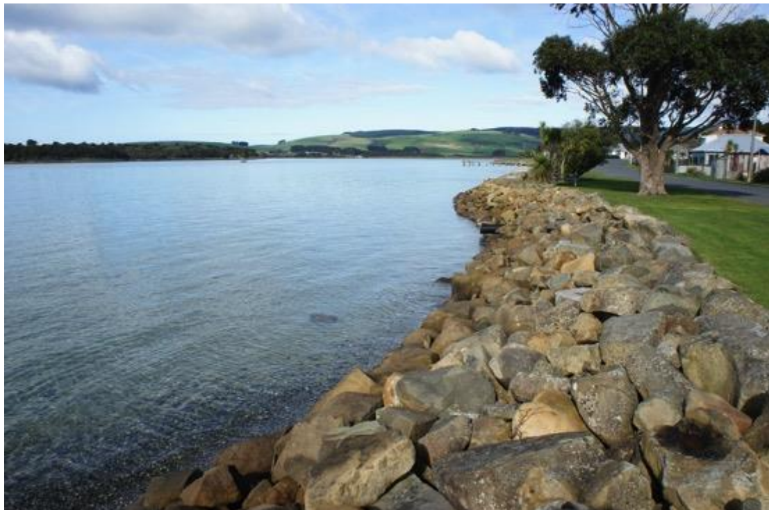
Figure 3-7 The Pounaweia sea wall (October 2019, Source: GHC).
