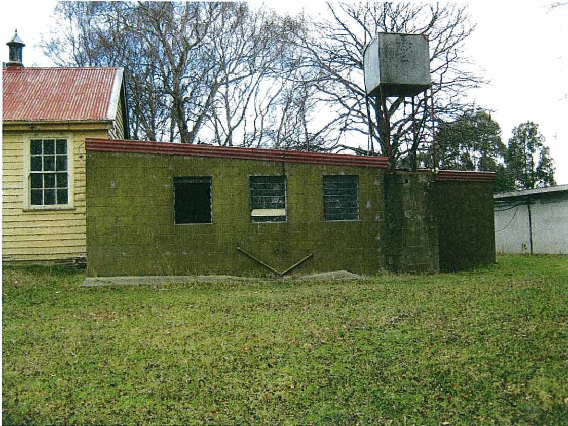
Concrete addition built in 1959.
