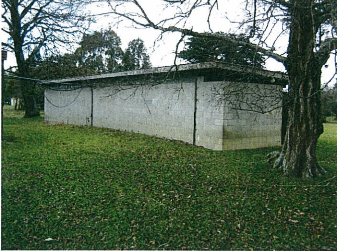
Existing Toilet Block at Tuapeka Domain Reserve
