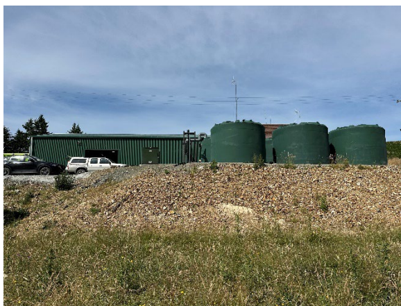
New Treatment Building and Clearwater Storage
