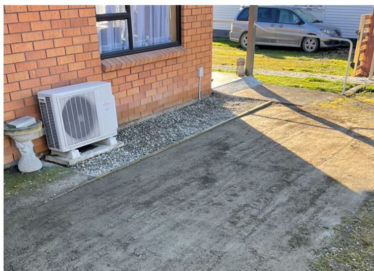
Work in progress for car park space
