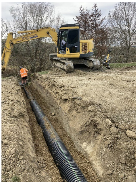
Culvert Replacement – Telegraph Road
