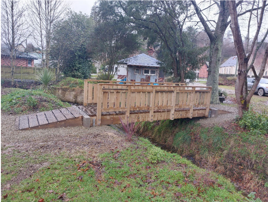
Fig 7: Lawrence Hospital Creek Timber Bridge
