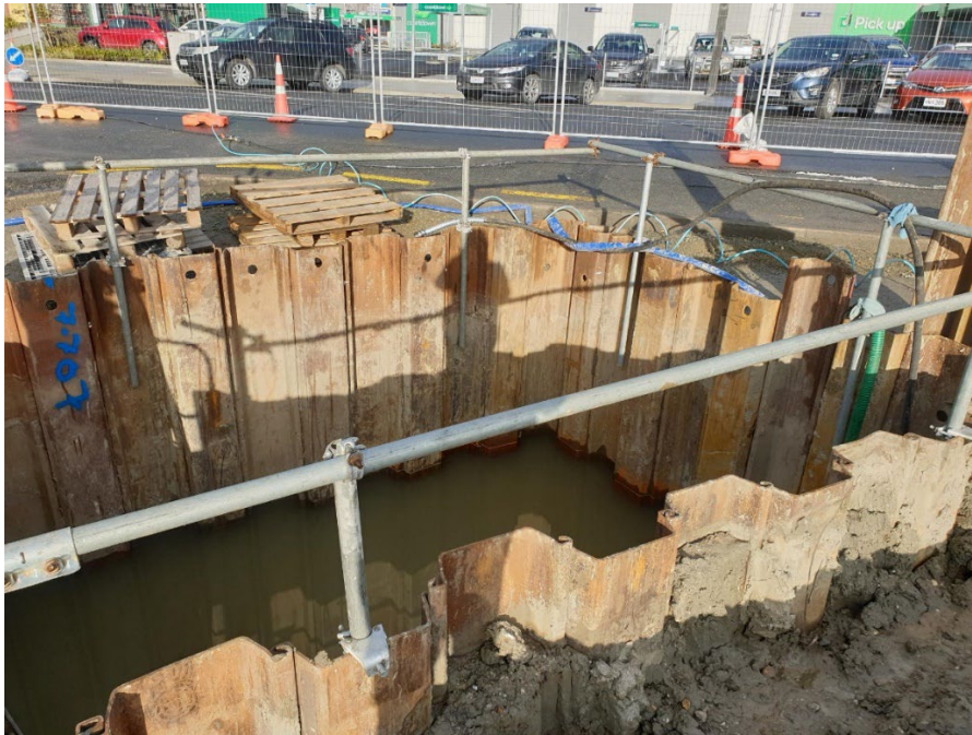
Fig 2: The Hub Wastewater Pump Station Sheetpiling
