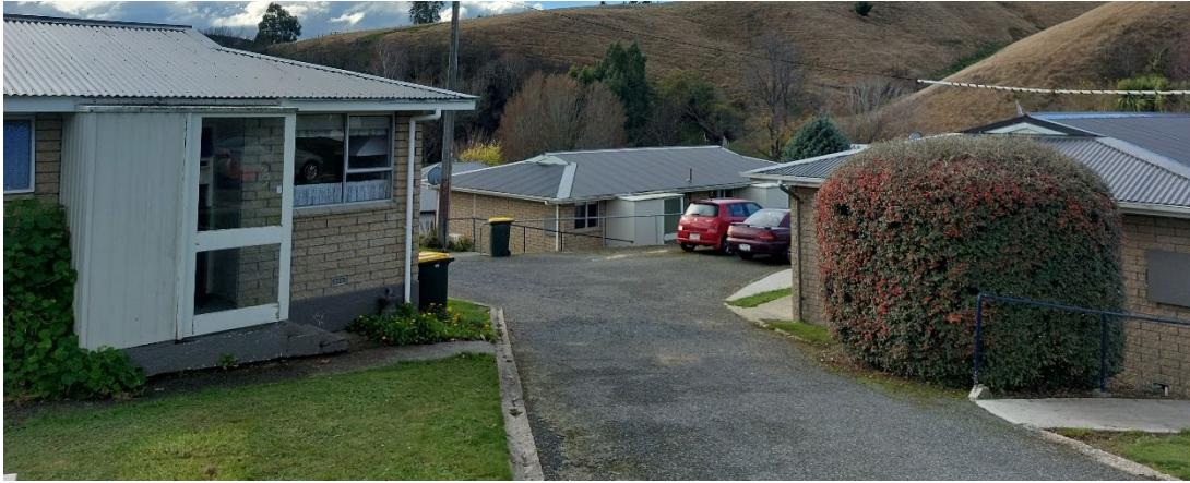
Fig 5: Lawrence Community Housing's new corrugated iron roofing.
