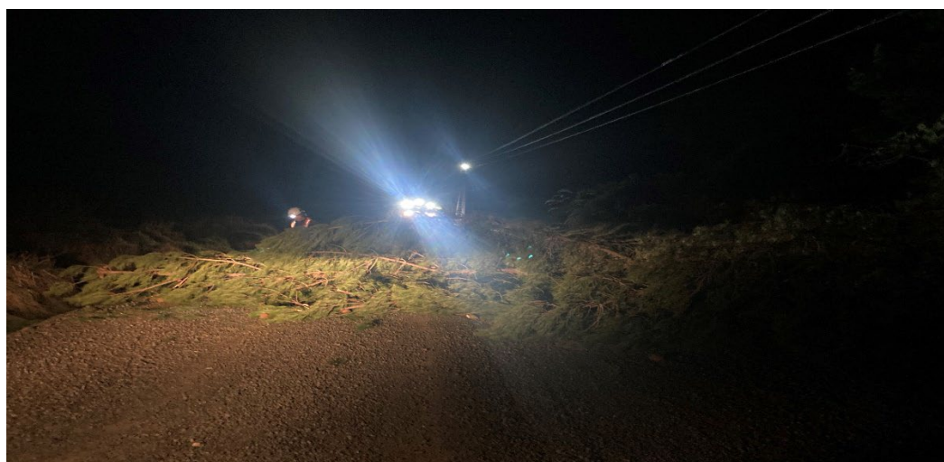
Clearing a fallen tree on Toko Mouth Road – 2.30am
