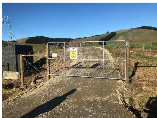
Waihola WWTP 1.8m deer fencing
