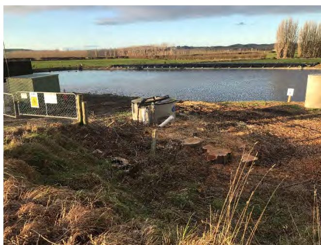
Stirling WWTP – Trees are removed preparing for Fencing work.
