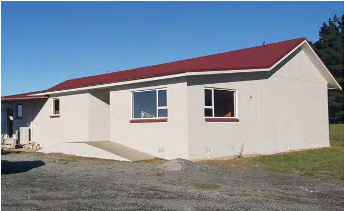
Figure 5 New roof on Hillend Hall.
