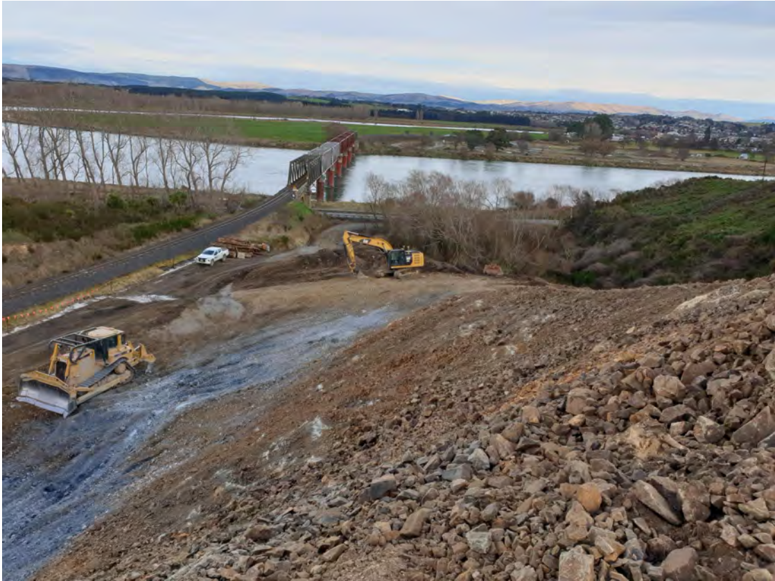
Figure 7 Work on Golf Course as part of stormwater diversion southern end.
