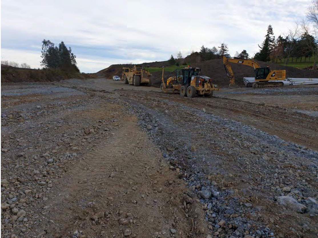
Figure 6 Work on Golf Course as part of stormwater diversion northern end.
