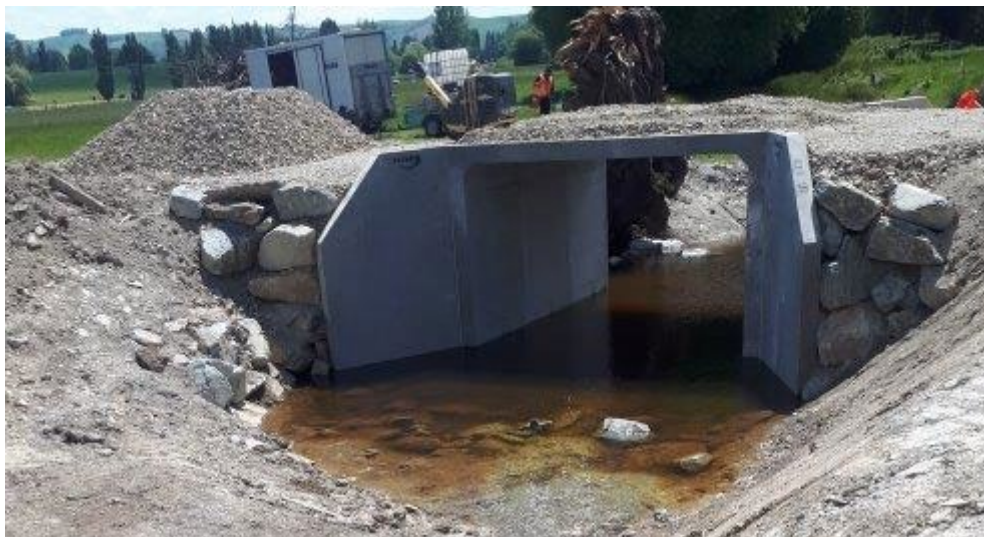
Figure 1 Ford Road box culvert
