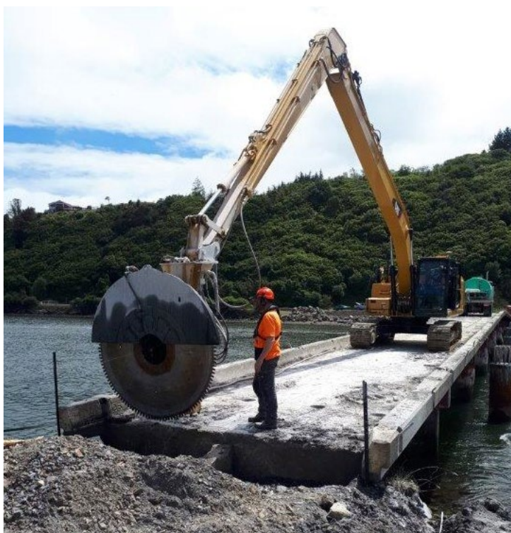
Figure Figure 2 Hinahina Bridge deck removal.
