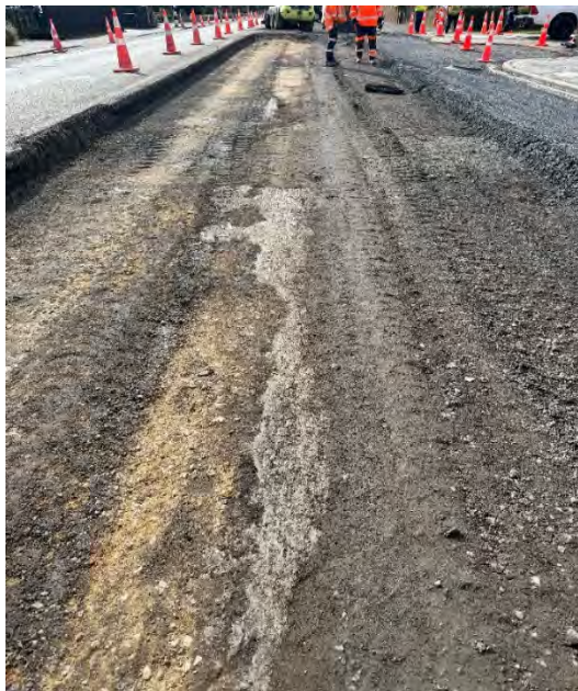
New Asphalt Union Street (Final surface SMA not installed)- After
