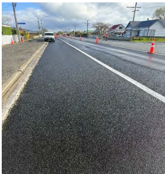
New Asphalt Union Street (Final surface SMA not installed)- After
