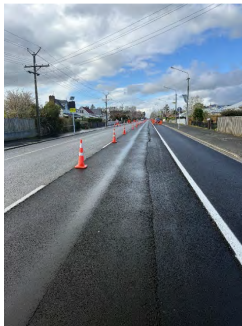
New Asphalt Union Street (Final surface SMA not installed)- After
