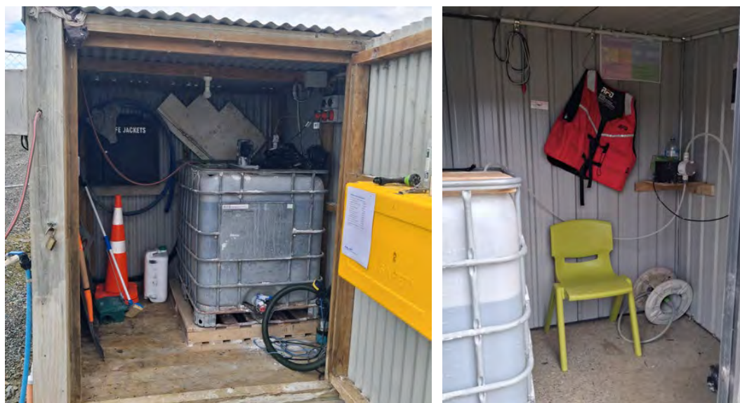
Stirling WwTP (l) and Tapanui WwTP (r) workspace sheds for operators showing lack of facilities
