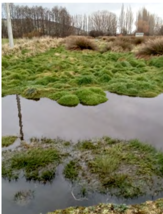
Milton Wastewater Treatment Plant – wetlands showing overgrowth and lack of delineation between cells
