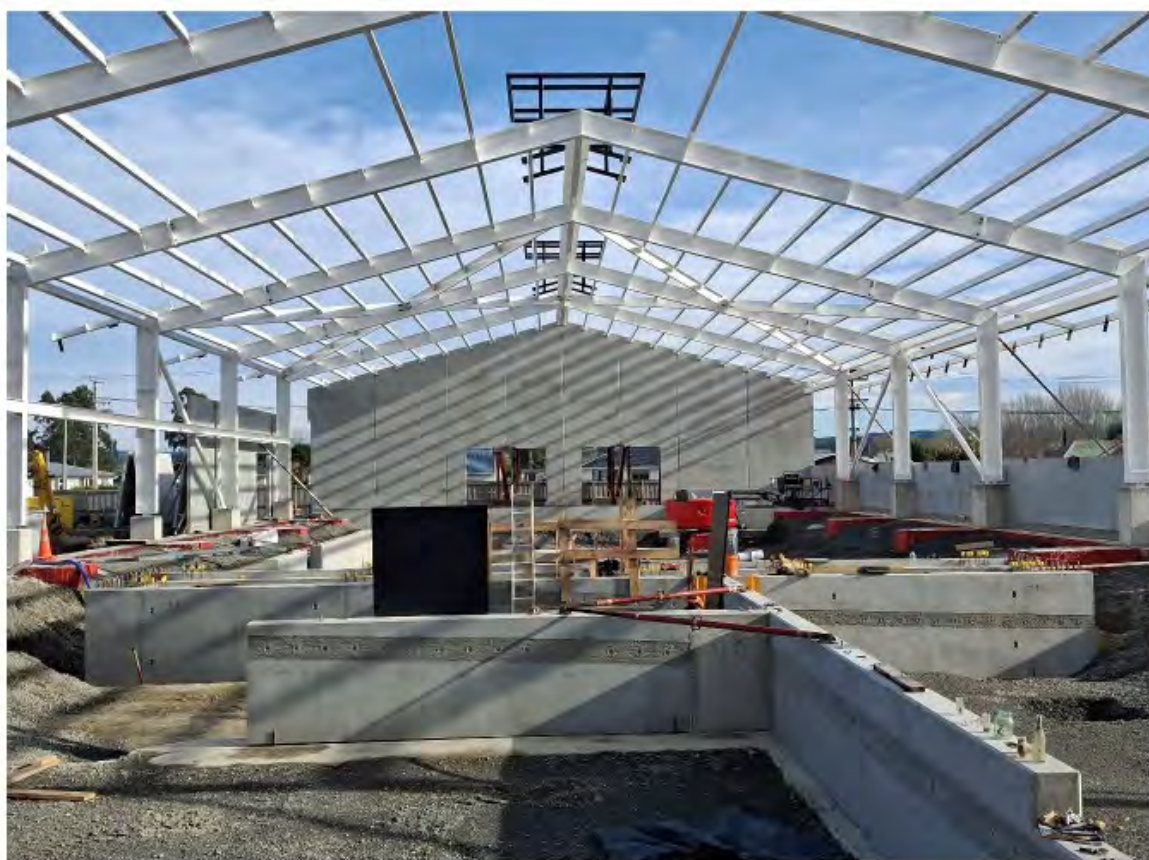
View of the pool panels from Grid 9
