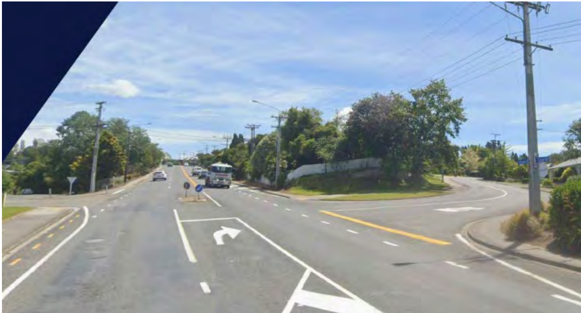
Figure 1. Existing SH1 Clyde Street Corridor at Rosebank Hill
