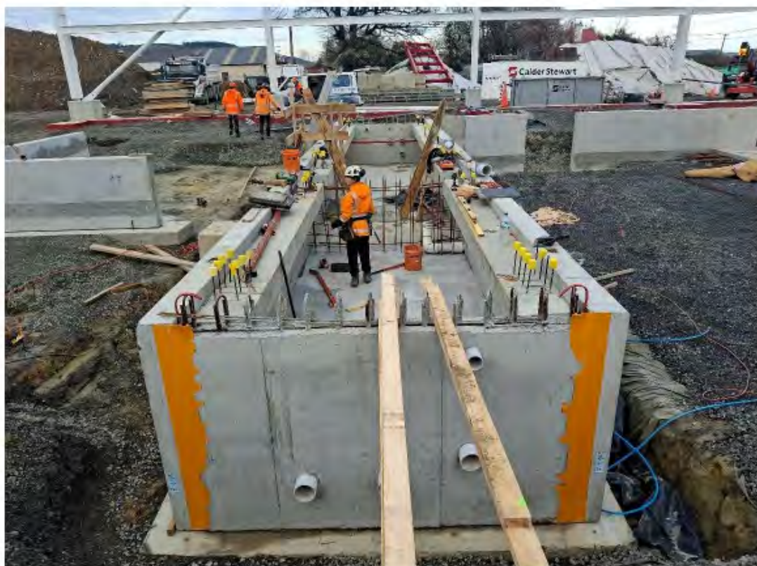
Balance tank progressing well
