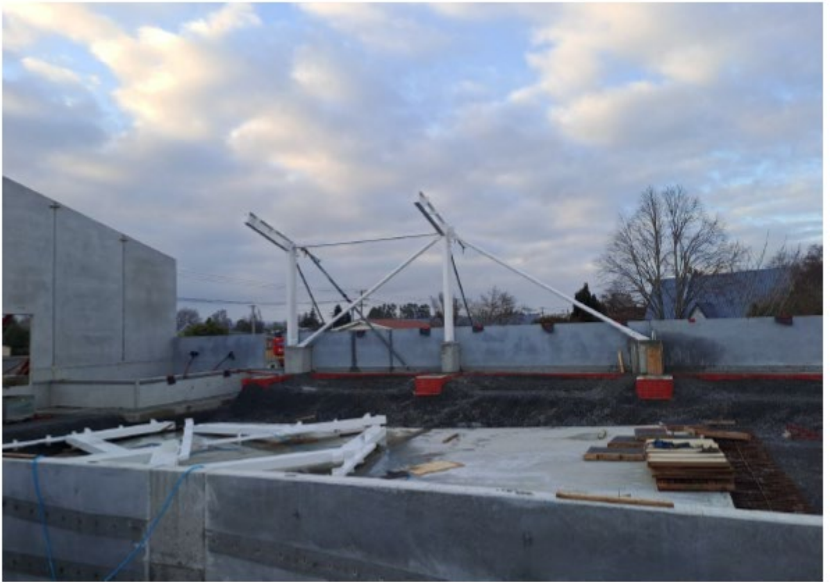
The first of the structural steel just erected
