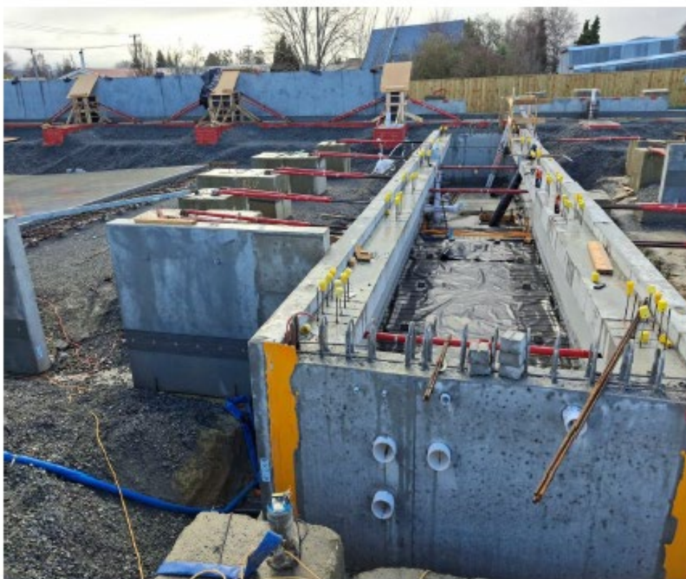
Balance Tank - preparations for slab base.
