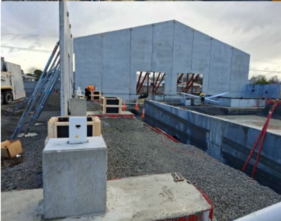
Concrete plinths to main pool hall progressing well.
