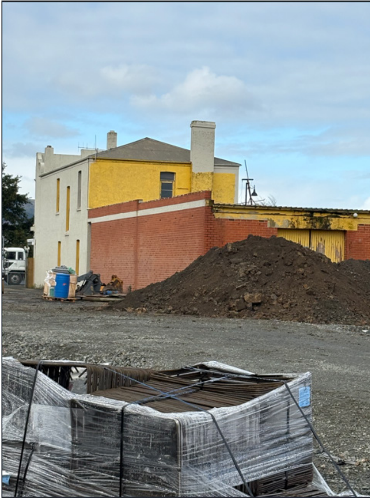
Back view of Building now owned by Calder Stewart that will be demolished
