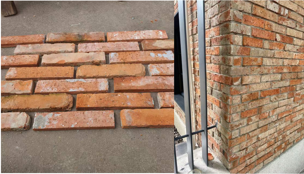
Photo 3. Brick venner sample (left), sample install (right)
