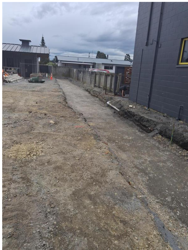
Photo 2. Preparation for the feature wall foundation (photo taken on 15 April)
