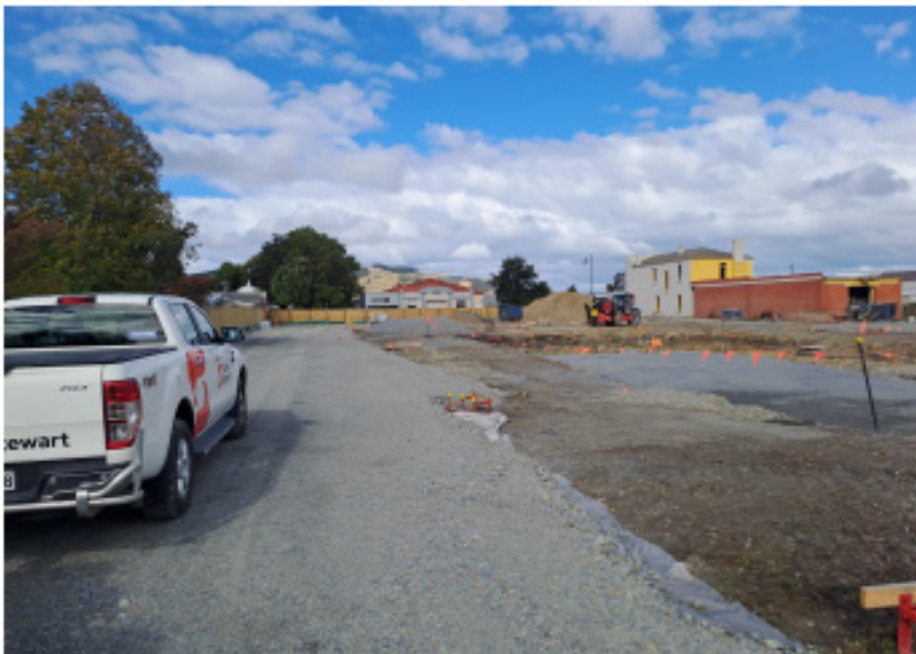
Eastern periphery looking tidy
