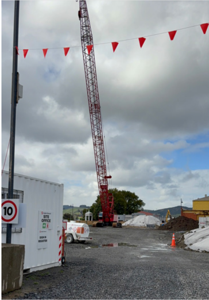
Large Crane now established on Site
