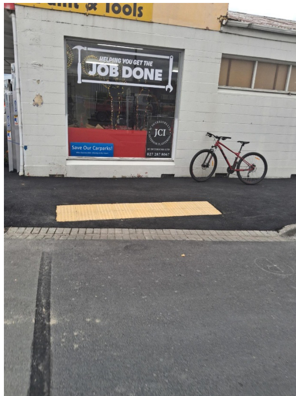
Photo 1. Footpath reinstatement (photo taken on 15 April)
