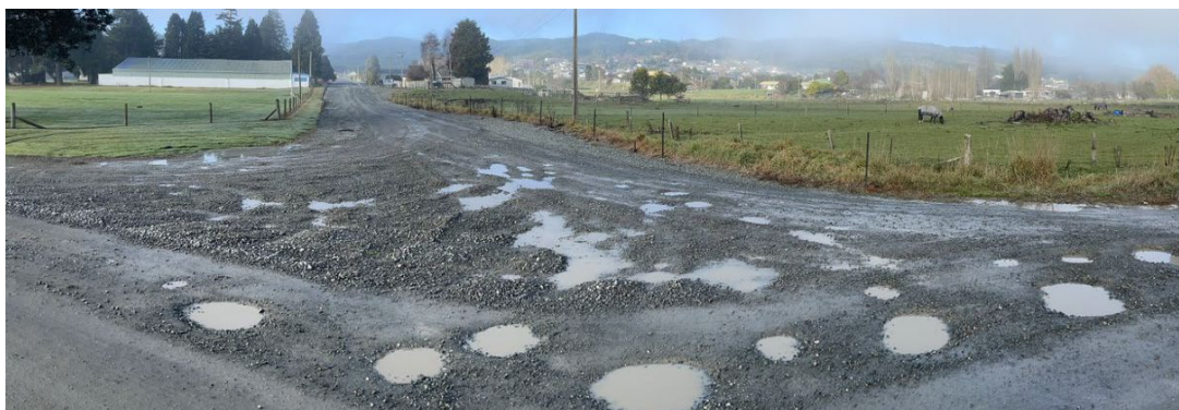
Figure 8. Intersection of St Albans and Water streets, June 2021.
