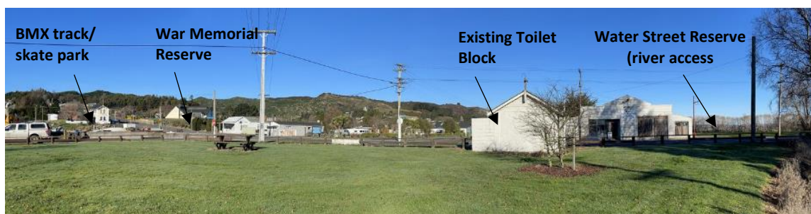
Figure 7. View of the old public toilet block on Exmouth Street, and adjacent facilities. June 2021
