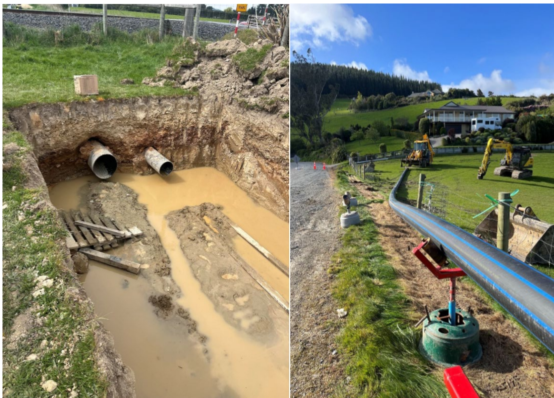
Bored Casing Pipes Ready for Pipeline Installation
