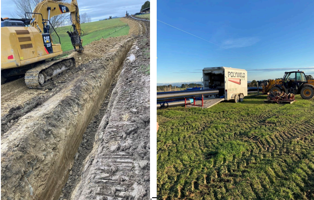
PE pipe being welded and Open pipe trench
