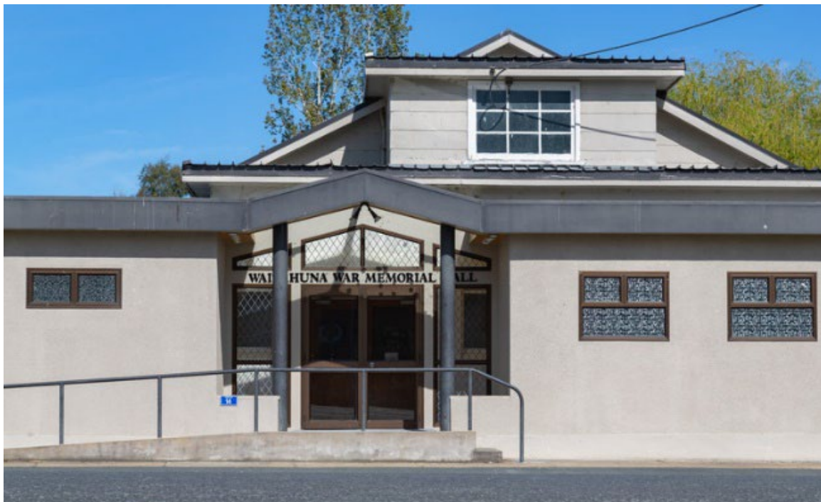
Figure 3 Exterior front view of Waitahuna War Memorial Hall
