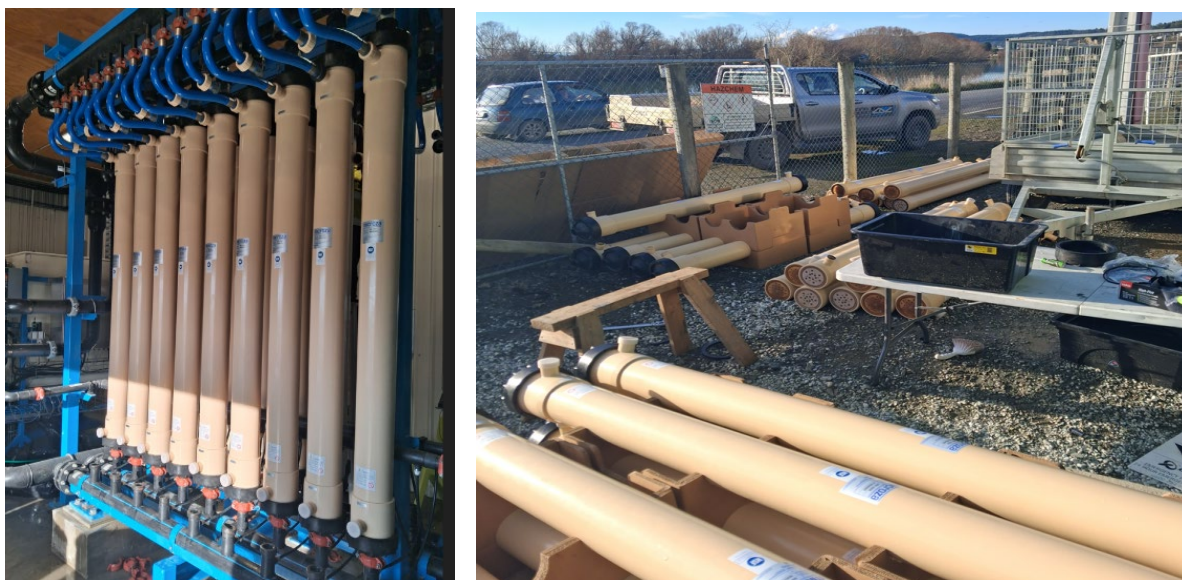
New membranes installed at Kaitangata WwTP
