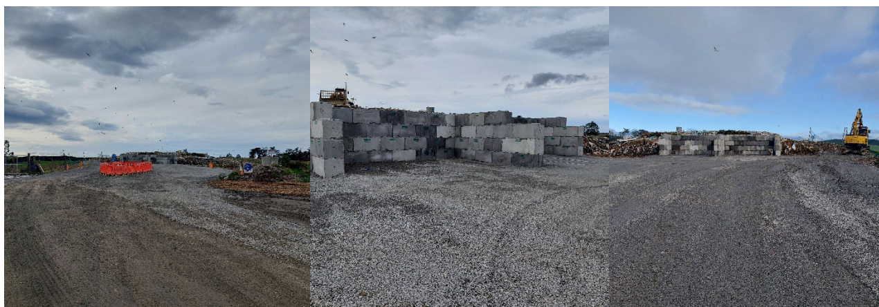
New transfer station
