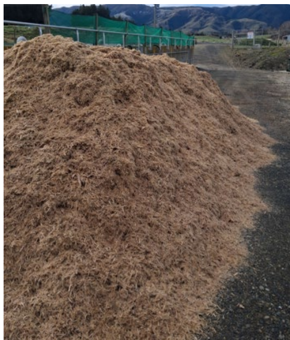
Tapanui WwTP – wood shavings ready to be added to raise the bed level
