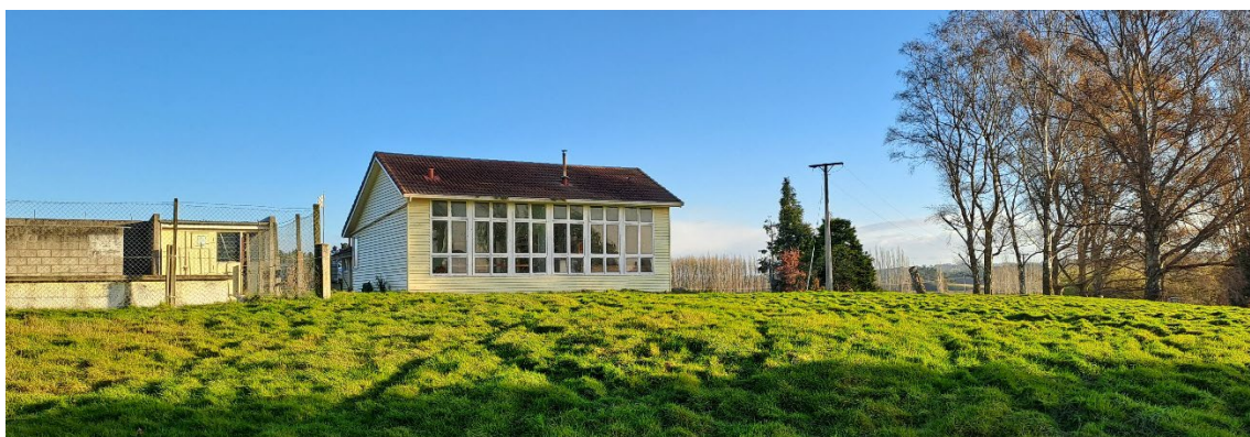
Figure 2 Lovell's Flat Hall, showing pool facility on the left (May 2026)
