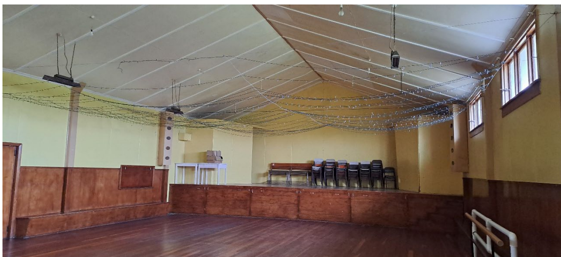
Figure 4 Interior view of Paretai Hall (June 2026)
