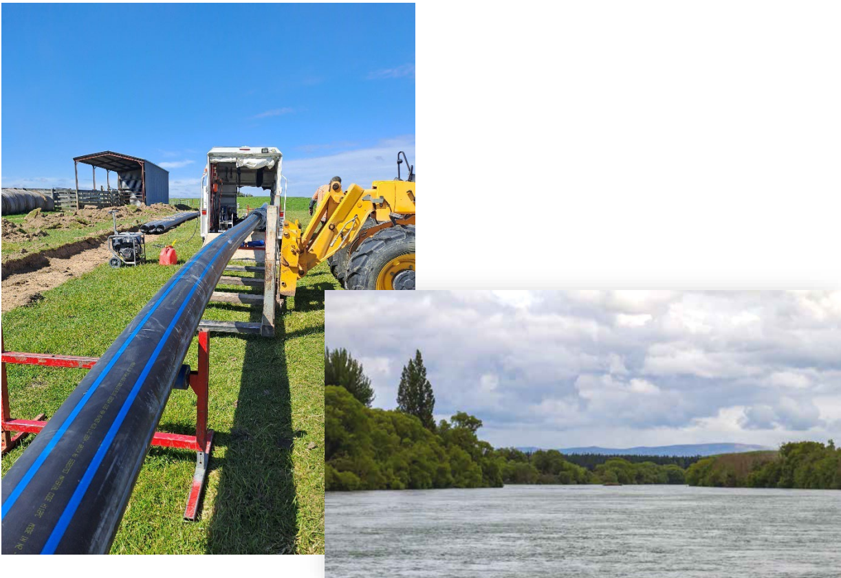
Figure 2-6 Pipe welding and installation (left) as part of the Greenfield Water Scheme Project which will link from the lower Clutha River (right) to Lawrence
