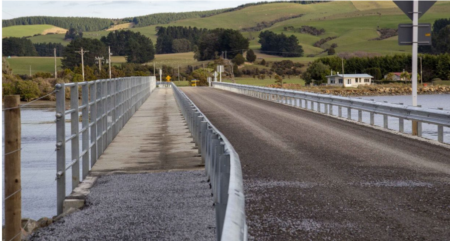
Figure 2-5 The new Hina Hina Bridge
