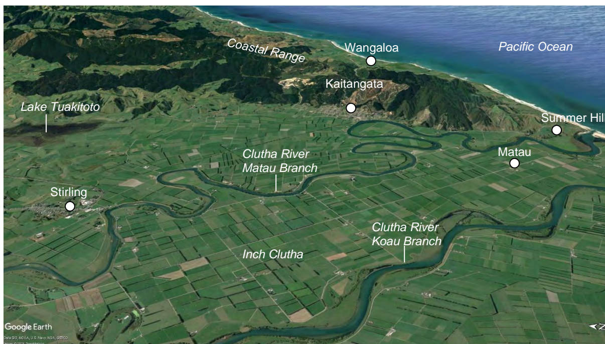
Figure 4-1 View to the east over the Clutha Delta towards Kaitangata and the Pacific coast (Google Earth)
