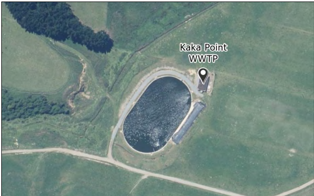
Figure 6.23: Kaka Point WWTP
