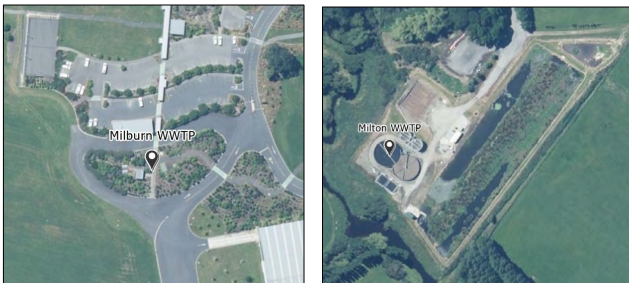
Figure 6.5: Milburn and Milton WWTP's
