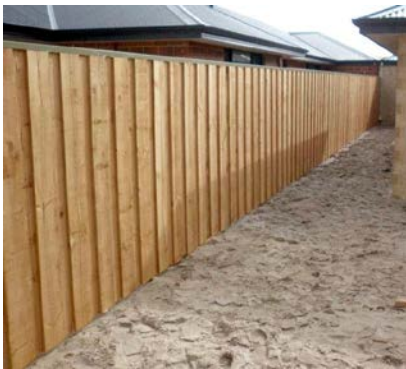
STYLE 1: Solid Timber Boundary Fences to the rear of the properties 2 metres high Oregon Place & 1.6m on Monterey Drive (pictured above)
