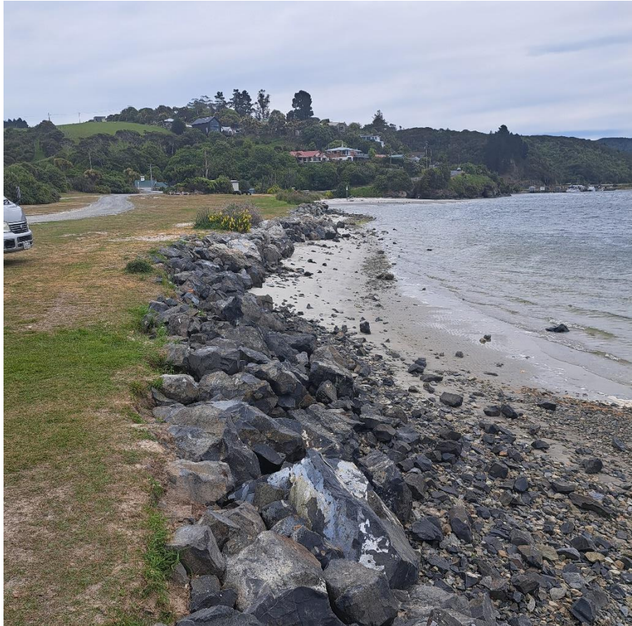
Figure 5-4 View of the riverbank at Knarston Park showing the grassed area, rock wall, and a mix of rocks and sand on the intertidal area.
