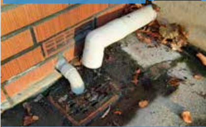
Non-Compliant gully trap
